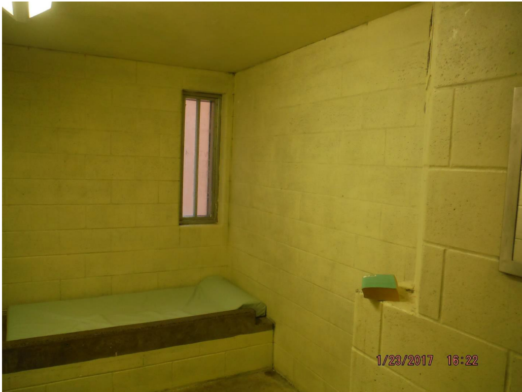
Figure 12 – Ottawa-Carleton Detention Centre Male Segregation Cell
