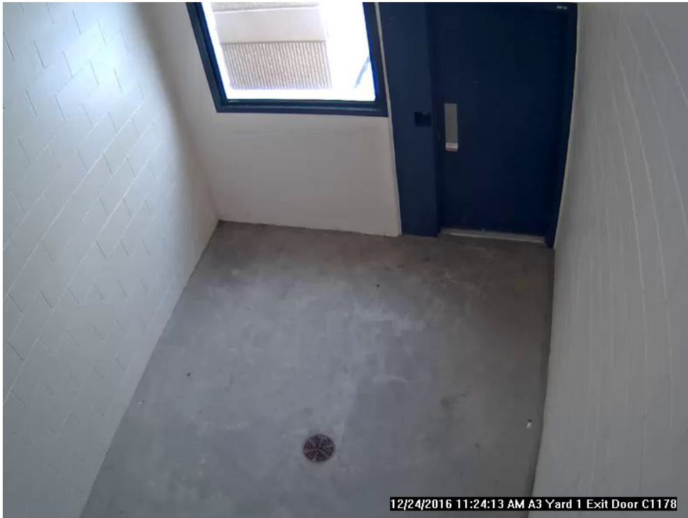
Figure 18 – South West Detention Centre Segregation Yard
