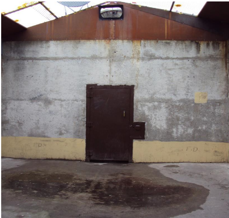
Figure 17 – Quinte Detention Centre Segregation Yard
