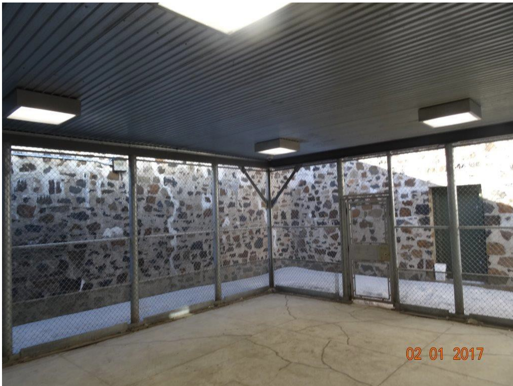
Figure 19 – Thunder Bay Jail Segregation Yard
