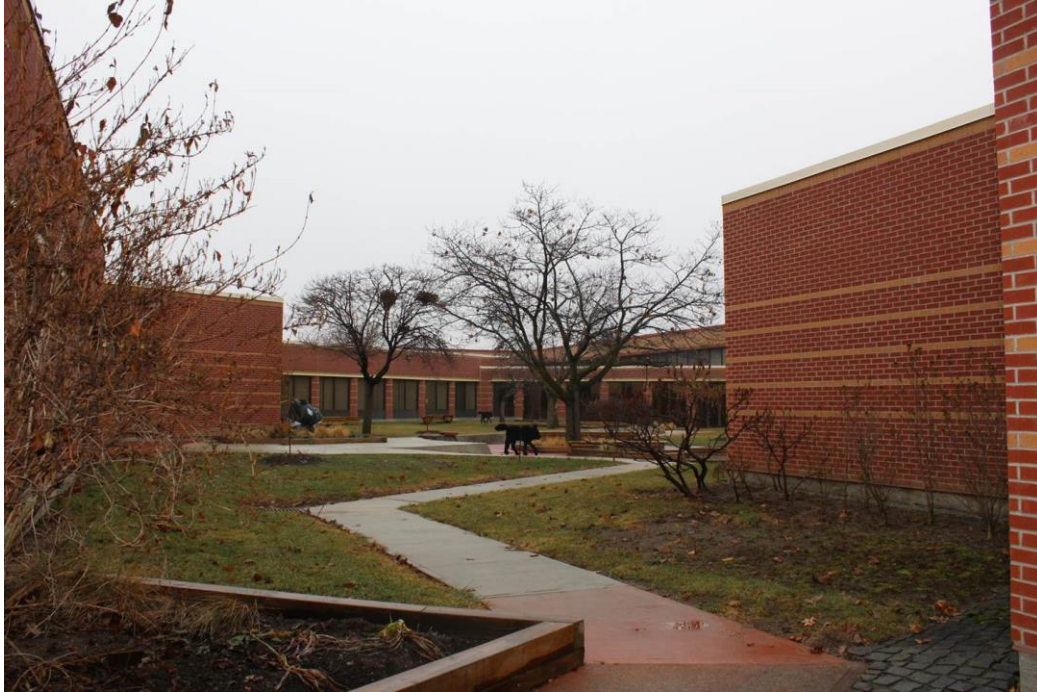
Figure 18: Yard, Ontario Correctional Institute
