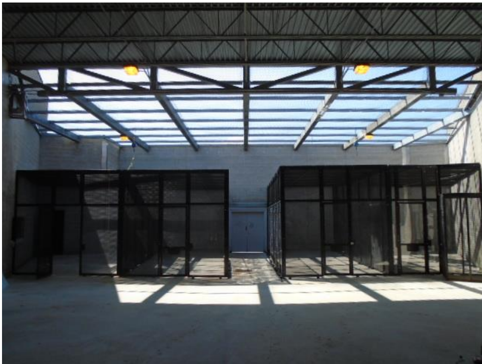
Figure 15: Step Down Unit Yard, Central North Correctional Centre
